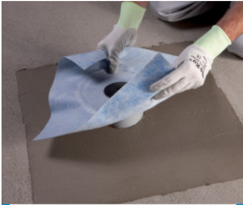
Application of Drain Vertical on Mapelastic
